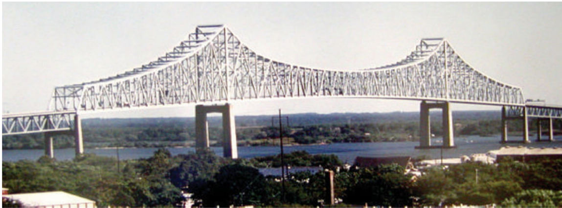
Fig. 42 An overview of the cantilever truss bridge [136]
