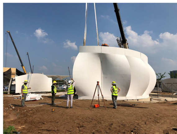
Fig. 2 2D Prefabrication showcase
