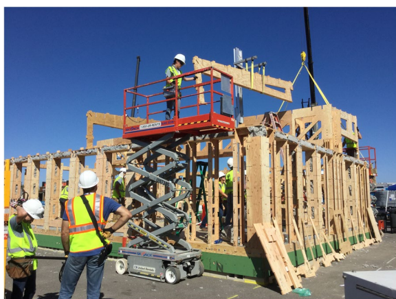
Fig. 1 1D Prefabrication showcase
