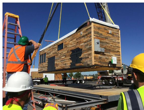
Fig. 3 3D Prefabrication showcase
