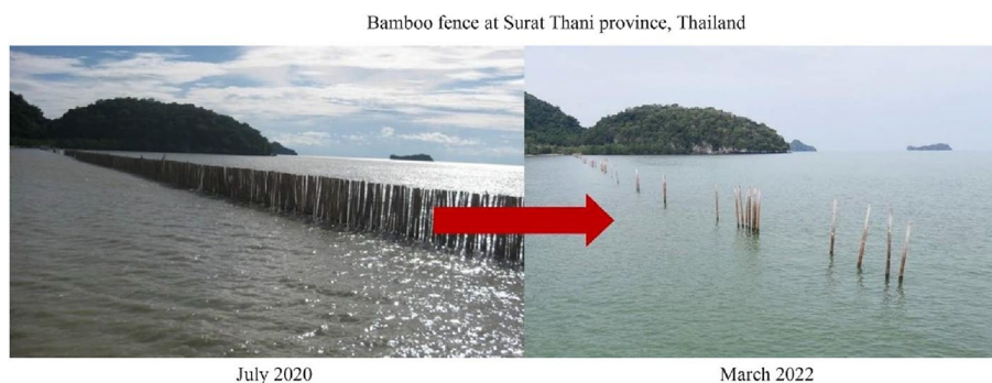
Fig. 2 Bamboo fences in Thailand
