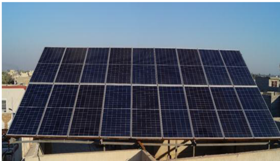
Fig. 1 Installation of the PV system
