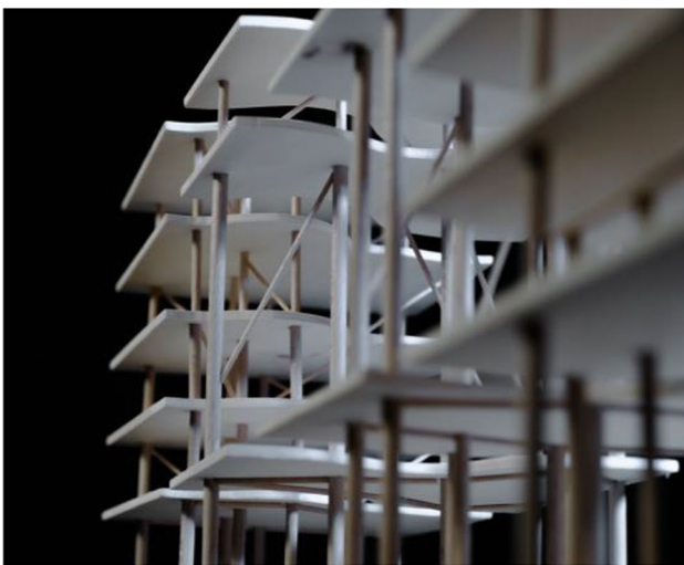
Fig. 9 The spatial openness of a structural strategy based on line structural elements, i.e. columns, permits large, continuous floor areas that may, or may not, be partitioned by non-loadbearing walls
