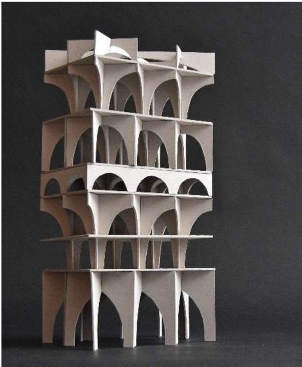
Fig. 15 Surface elements as walls with large cut-outs. Project and model by Edward G. Wahlström Nesse and Maria Højgaard Molden. Photo; Joar Tjetland
