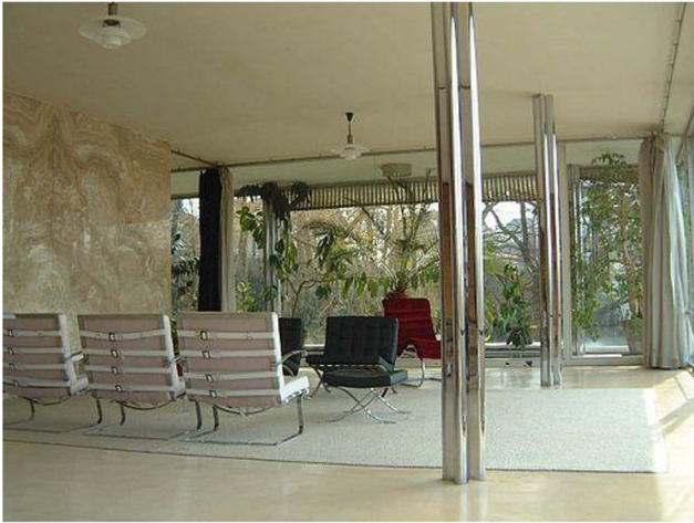
Fig. 8 The modernist Tugendhat House shows a skeletal system of columns that enable space to “float” unrestricted in-between. Photo; Wikimedia Commons/User: Simonma
