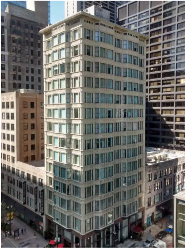
Fig. 2 The highlight of the Chicago School, the Reliance Building from 1895 by Burnham and Root, and architect Charles B. Atwood, with E. C. Shankland as lead structural engineer. Photo; Wikimedia Commons/Mx. Granger
