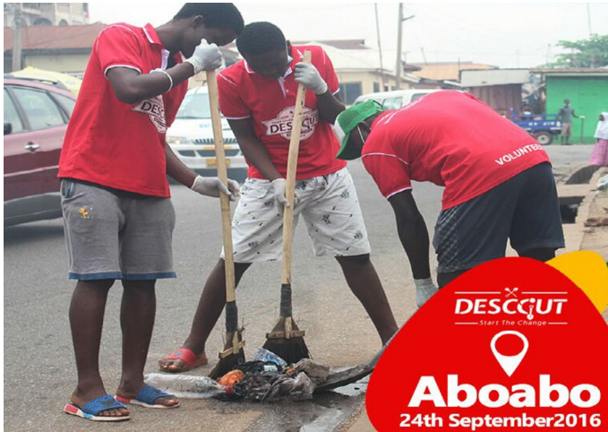
Fig. 5 Descgut desilting of choked gutters in Aboabo
