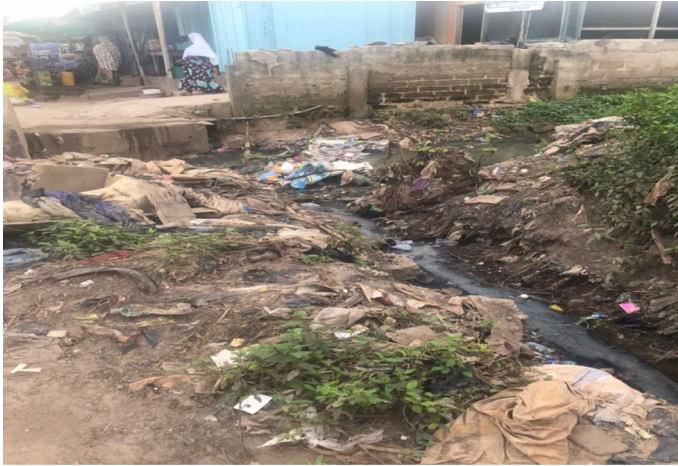
Fig. 2 Poor sanitation and solid waste management in some parts of Sawaba. Source: Field Survey, July 2021
