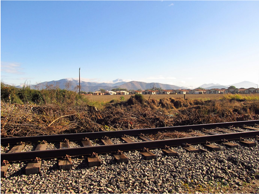
Fig. 7 Railway lines in the conurbation between Santiago and Padre Hurtado. At the back, farming spaces and new social housing developments (author's photo 2014)
