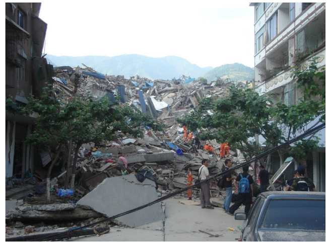
(b) Overall collapse
