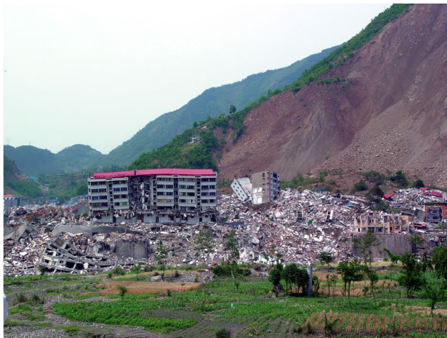
(a) Overall failure of the building cluster
