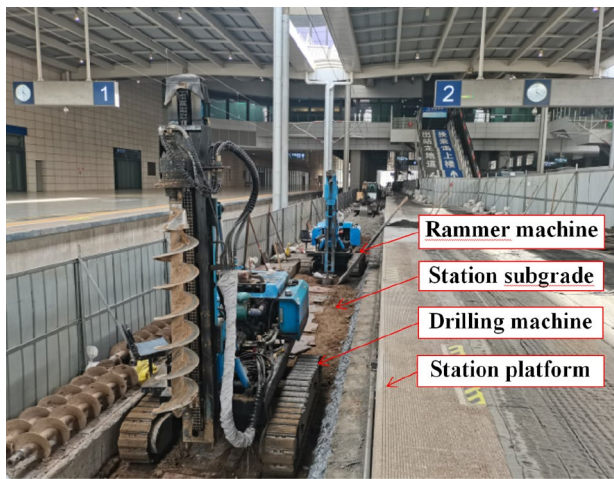
Fig. 1 Pile drilling machine and rammer machine
