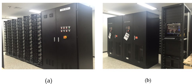
Fig. 10 Demonstration PCS and ESS at site #2, a Lithium-ion ESS (571.8kWh); b PCS (500 kW)
