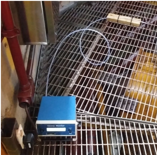
Fig. 19 Ozone monitoring in the generator-motor room
