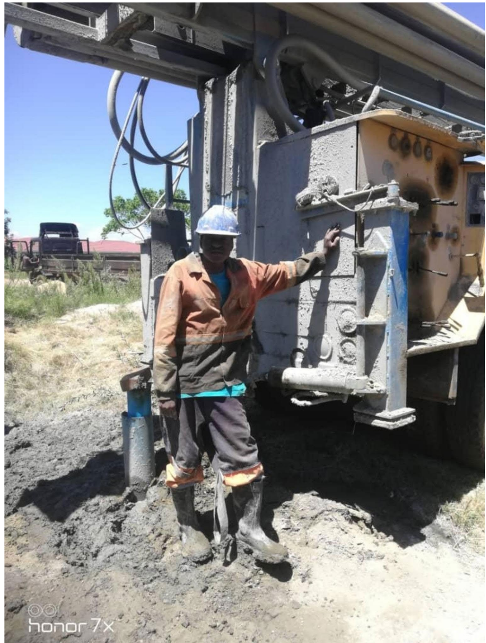
Plate 1 A worker without adequate PP/C. Source: field survey (2023)
