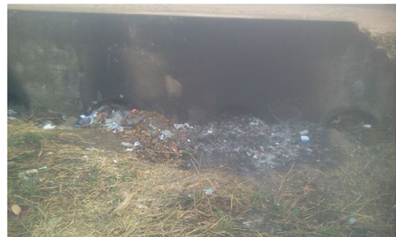
Plate 1 Solid waste in and around drains. Source: Authors (2023)
