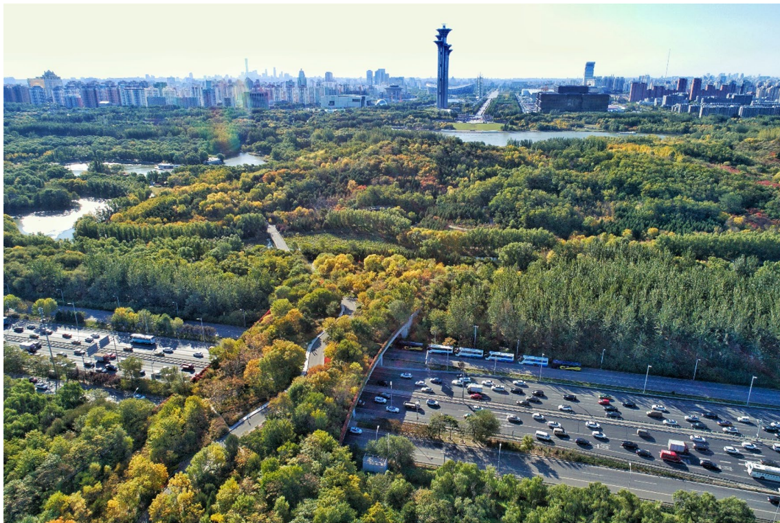
Fig. 4 The eco-bridge across the North Fifth Ring Road connects the north and south park (Fall 2019). Source: THUPDI; used with permission
