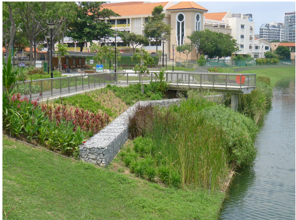
Fig. 5 A waterway enhancement project at the Kallang River at Potong Pasir in Singapore. Several lookout decks were installed at the river bank to allow people to be closer to water. The river bank was made greener with lush and diversified vegetation to improve aesthetics
