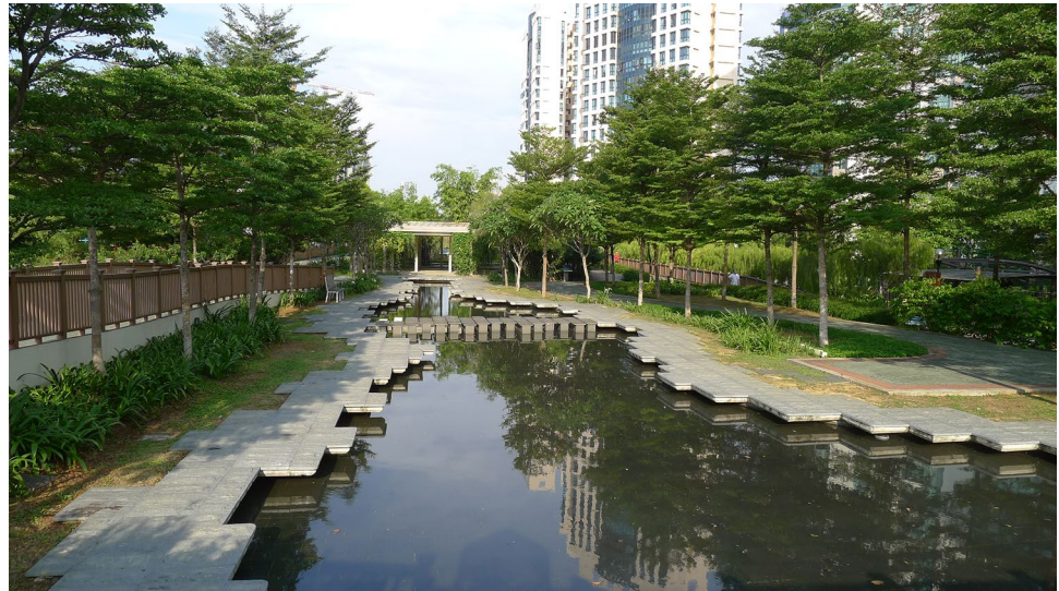
Fig. 8 The community space at the Alexandra Canal in Singapore, as a waterway enhancement project in the ABC Waters Program, was created through decking over a section of the canal
