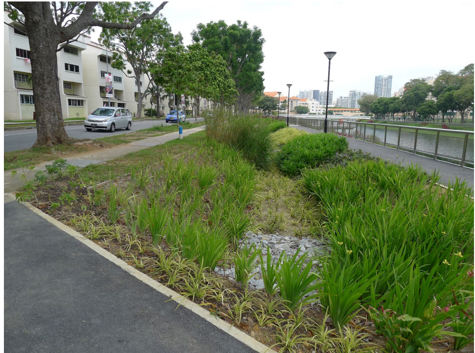
Fig. 3 A bioretention swale near the Kallang River at Potong Pasir in Singapore
