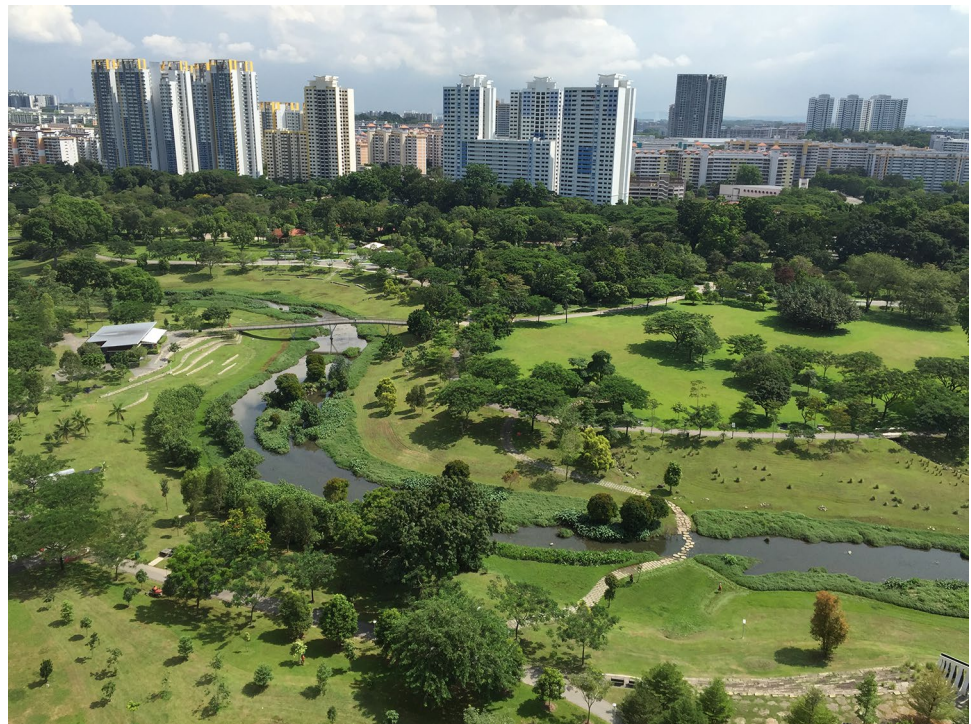
Fig. 6 The Bishan-Ang Mo Kio Park, where the naturalized Kallang River is integrated with its surrounding terrestrial green space
