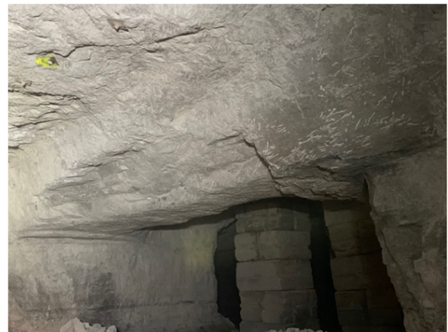
Fig. 5 Example of partial failure of a full window
