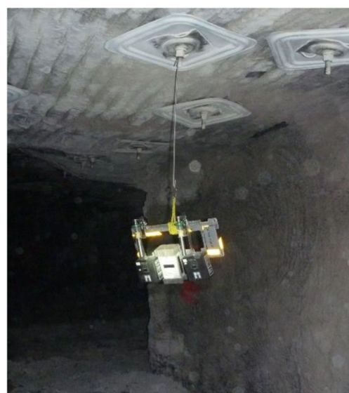
Fig. 3 A typical sampling package consisting of a pDR and two gravimetric samplers. This package is typically hung from a roof bolt
