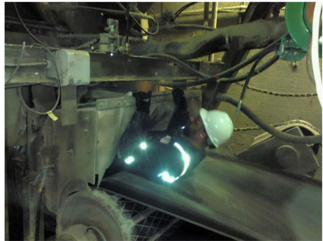
Fig. 1 Entering mixer drum to perform maintenance
