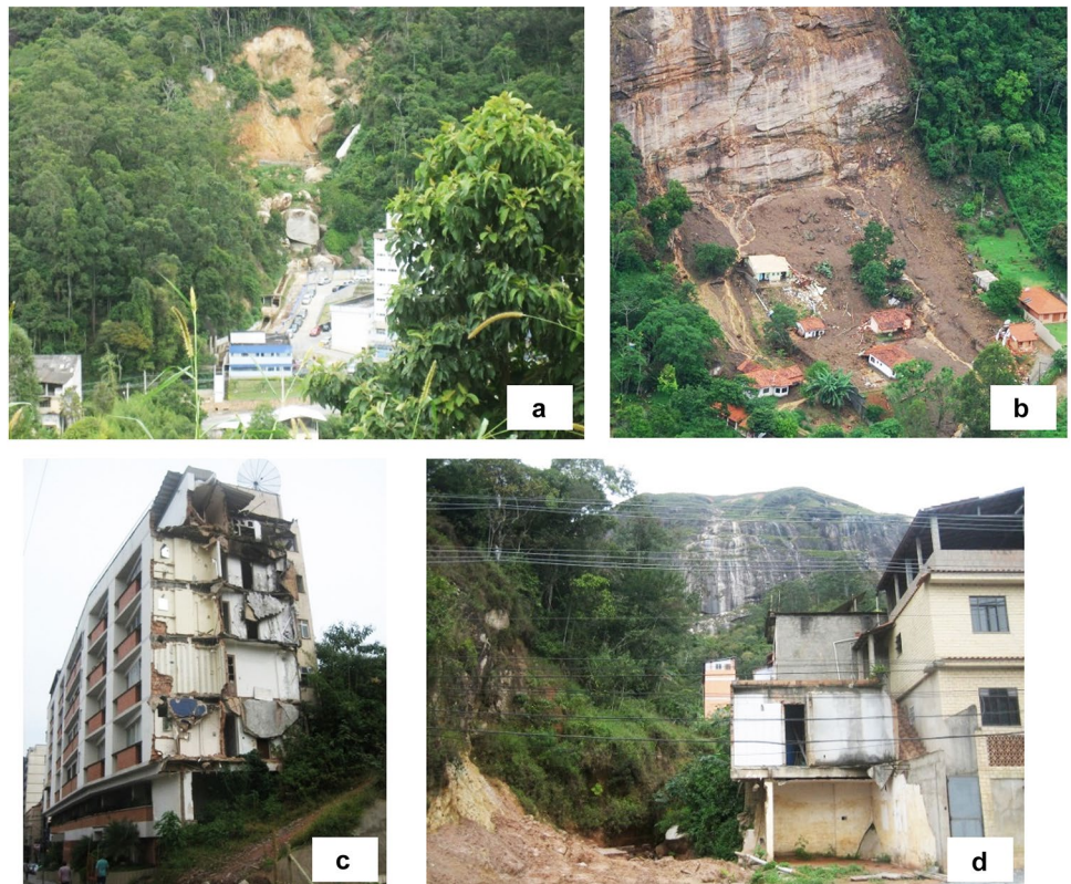
Fig. 15 a Rock blocks at the base resulting from a landslide; b Nova Suiça. Planar landslide with material deposition; c building destroyed by a landslide; d building partially destroyed by a landslide
