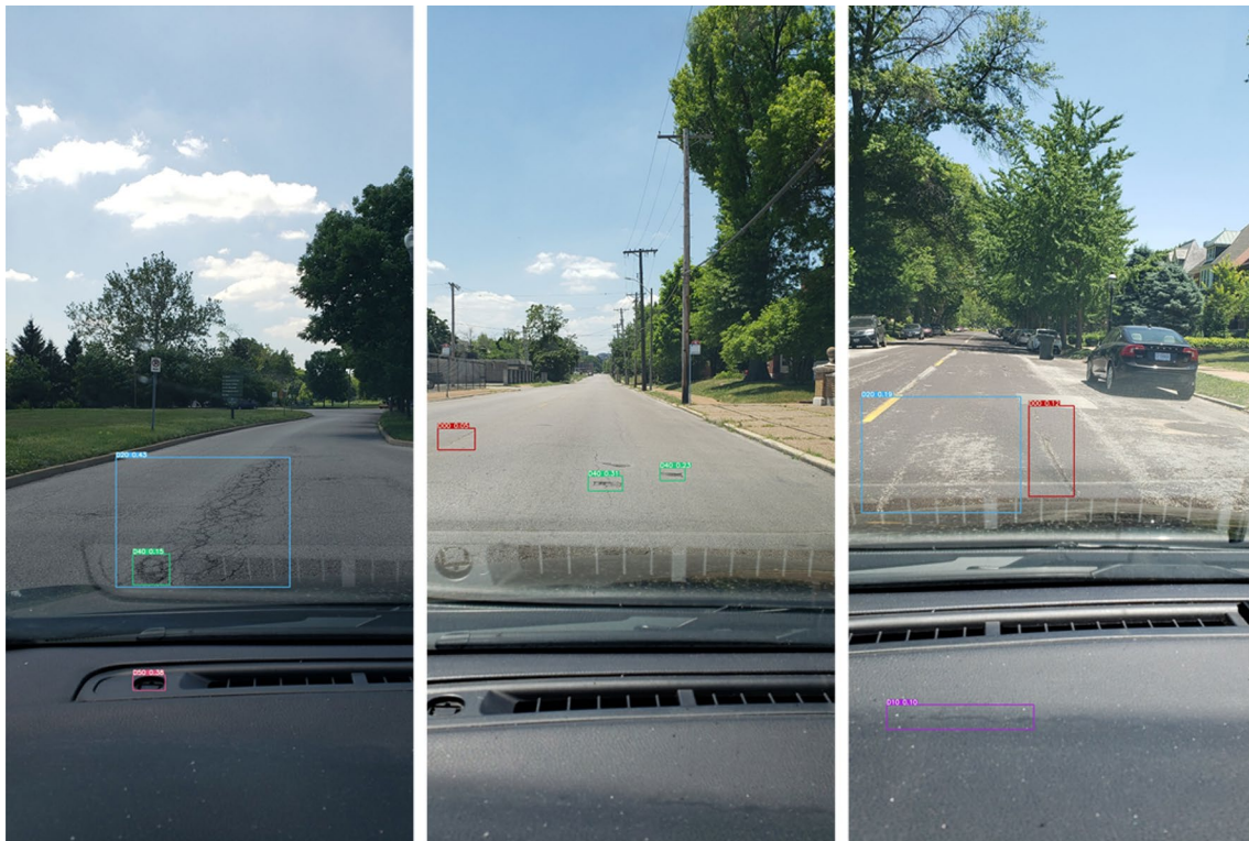
Fig. 11 Pavement distresses detected from video data
