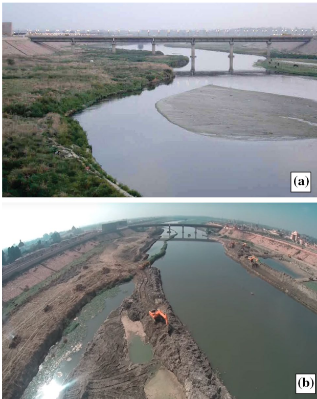
Fig. 8 a Heterogeneous habitat patches with sand bars and river pool during year 2011. b Loss of channel width and channel connected pool during the channelization project in 2015
