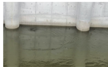
Fig. 1 (Color online) Picture of an inlet vortex
