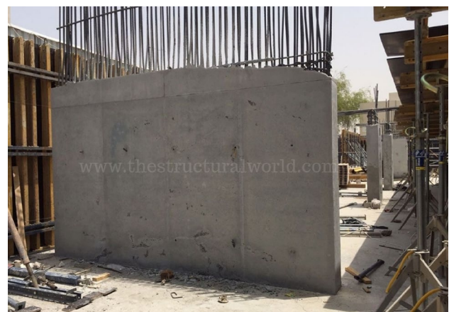
Fig. 1 Shear wall (Source; www.constructionworld.com )
