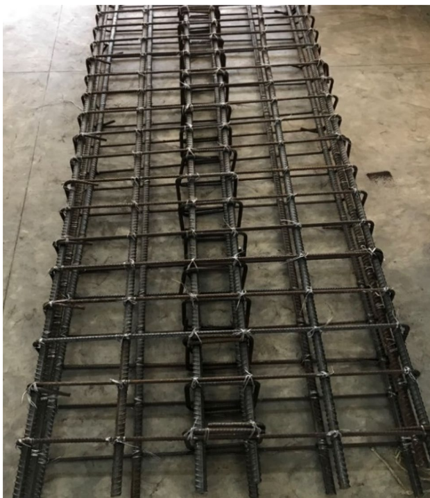
Fig. 6 Reinforcement arrangement for base slab
