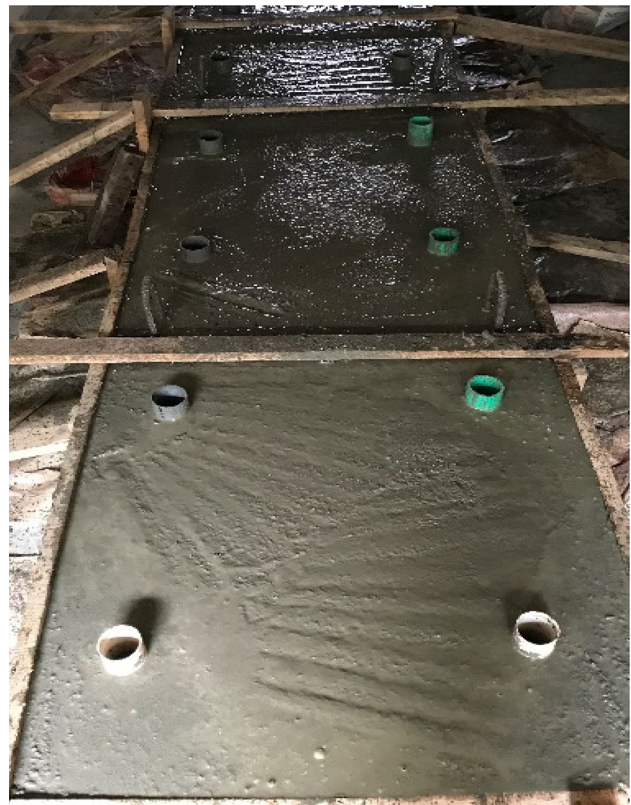
Fig. 7 Base slab after casting
