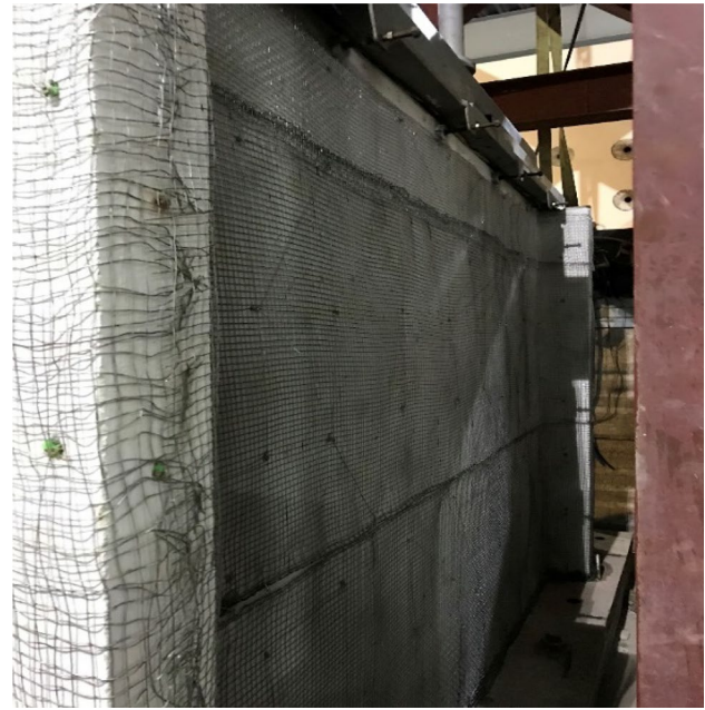
Fig. 9 Wire mesh on plastered wall
