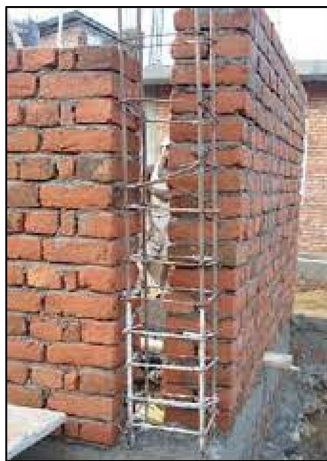
Fig. 12 Confined Masonry Wall
