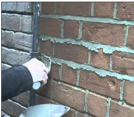
Fig. 7 Repointing Technique
