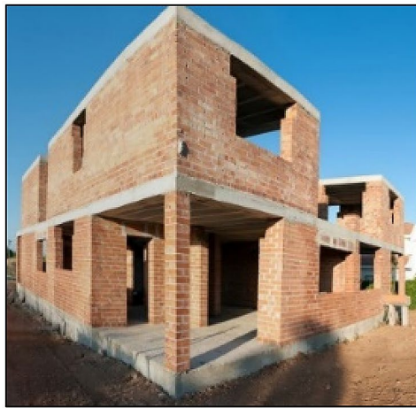
a Load-bearing wall
