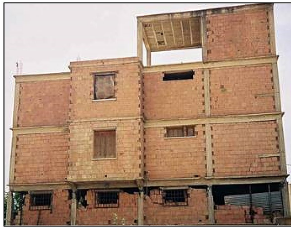
b Non-load-bearing wall
