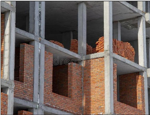
Fig. 11 Masonry Infill Wall
