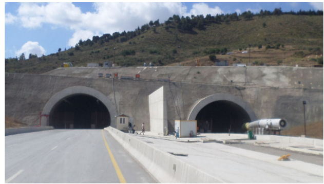
Fig. 1 General view of two tubes of tunnel T1
