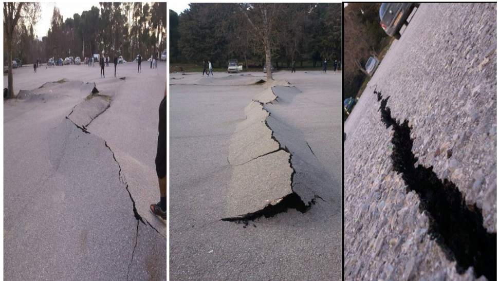
Fig. 6 The state of place of the structure after the collapse (lifting of ground above left tunnel, and destruction of roadway)
