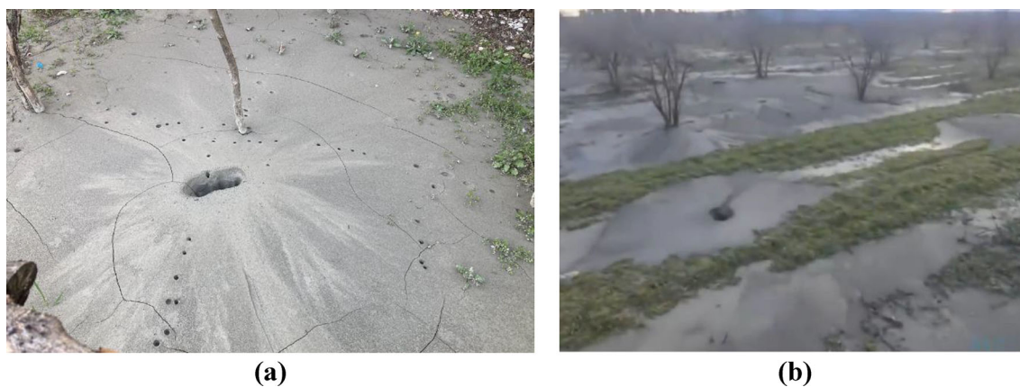
Fig. 1 After the Turkey–Syria earthquakes (2023): a liquefaction at the edge of Hatay city, and b soil liquefaction in northern Syria (Gazetas and Garini 2023)
