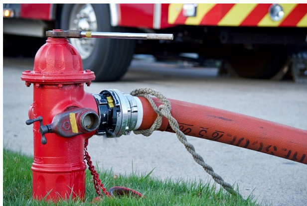
Fig. 4 During the fire incident, a fire hydrant was connected to a hose. (Courtesy: Shutterstock)
