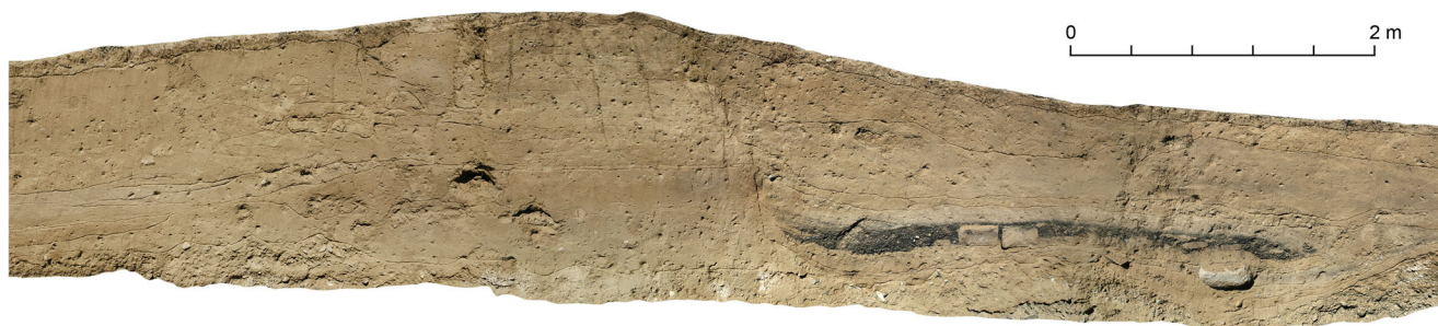
Fig. 7 Section through the northern part of the outer city wall of Karakorum. The section is located nearby the assumed northern main gate to the northwest, taken in 2014 (photo © Bonn University, used with permission)
