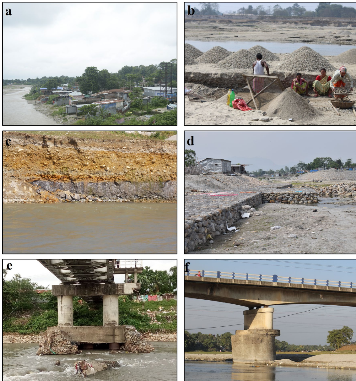
Fig. 8 Evidences of anthropogenic stresses and its impact on Balason and Mahananda River; a Encroachments of a point bar found on Mahananda River bank at Champasari; b Large amount of sediment is getting withdrawn from Balason River bed at Matigara; c Ground water is getting discharged from exposed water carrying layer as a result of bed lowering on Balason River at Tarabari; d Heavily
