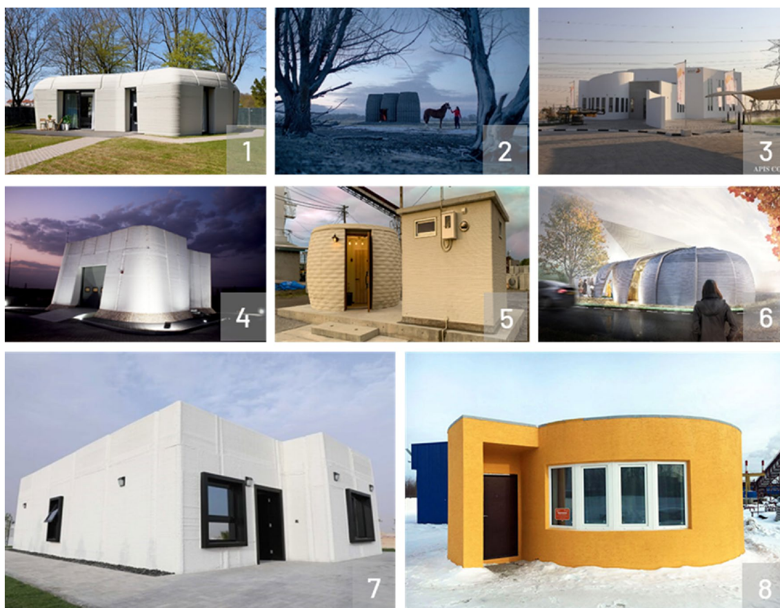
Fig. 8 (1) Eindhoven house (Parkes 2021a), (2) Casa Covida (Block 2021), (3) Dubai municipality (Harrouk 2019), (4) Dubai drone laboratory (CyBe 2017b), (5) Toilet units (CyBe 2020), (6) House in the
