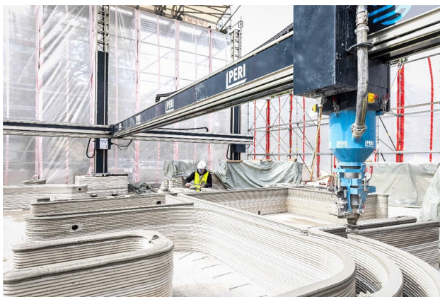
Fig. 1 Printing process with the BOD2, source: PERI
