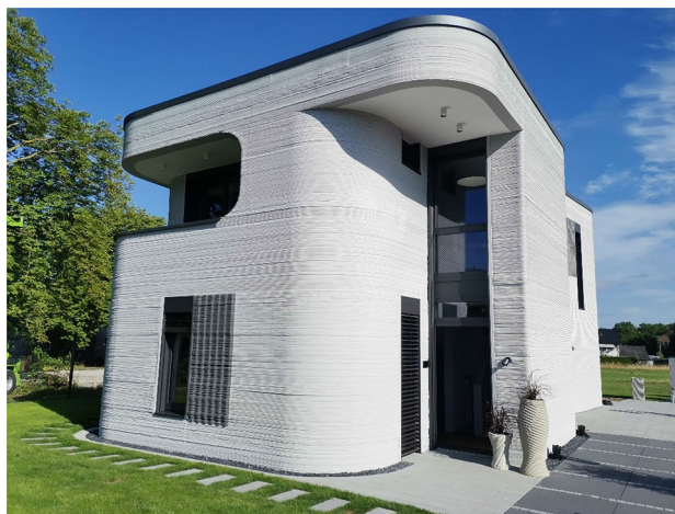
Fig. 10 Germany's first 3D-printed building, source: HeidelbergCement Group
