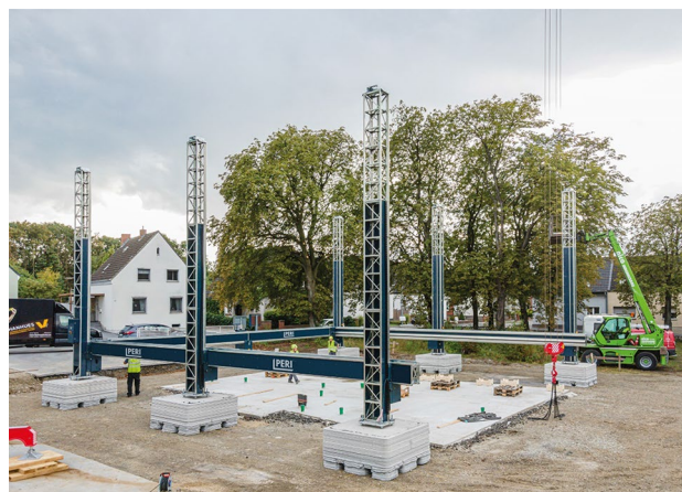
Fig. 8 Assembly of the COBOD BOD2 3D concrete printer
