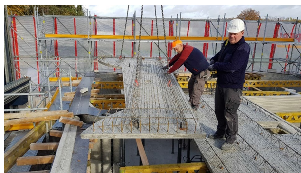
Fig. 5 Construction process with suspended ceiling, source: MENSE-KORTE
