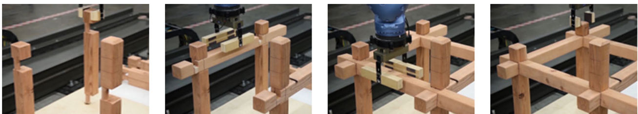
Fig. 5 Sequence of joint assembly: part A (a), part B (b), part C (c), the final twist to lock everything in place (d)
