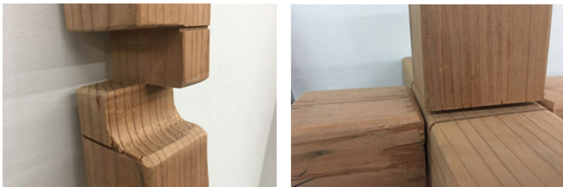
Fig. 3 Details of the chamfered edges for tolerance (a) and the assembled joint with the tolerances (b)
