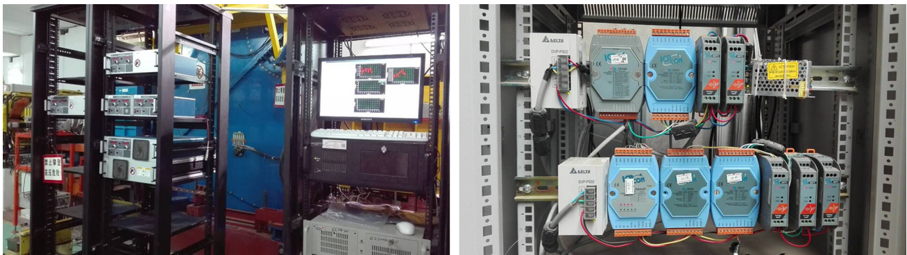
Fig. 2 Hardware setup of electronic cooler system for CSRm
