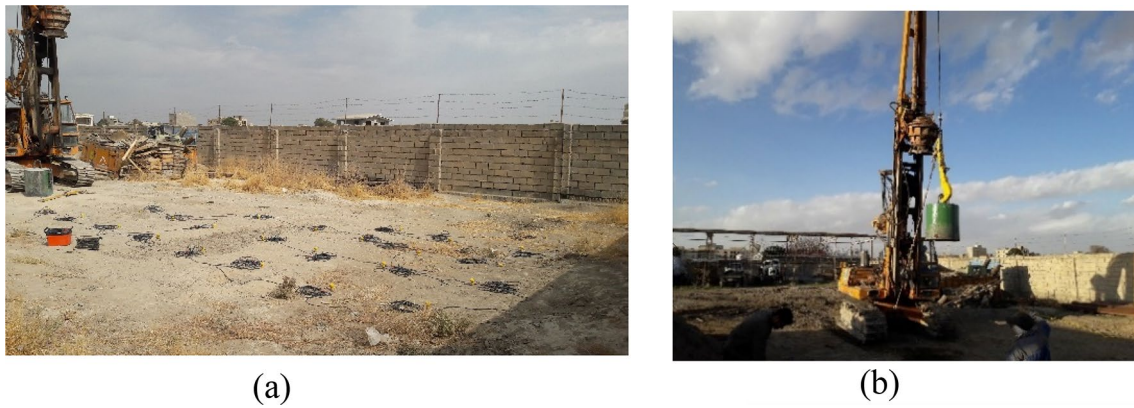
Fig. 5 Images of: a installation of geophones in ground; b falling dynamic compaction tamper
