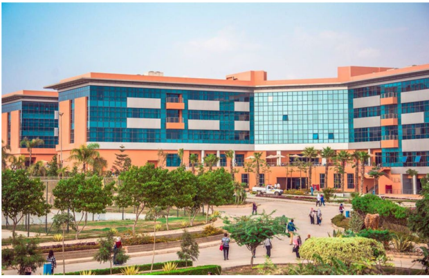
Fig. 3 D-building in the German university in Cairo
