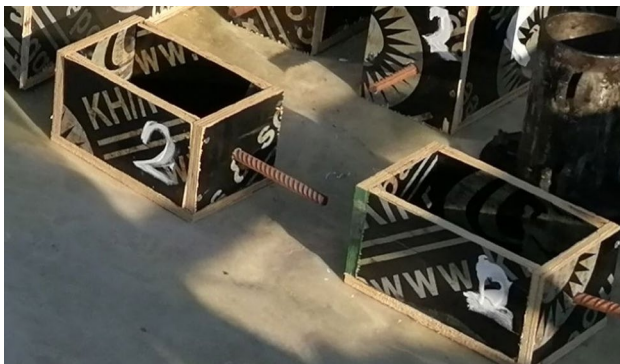
Fig. 5 The wooden molds are ready for casting the lightweight concrete blocks
