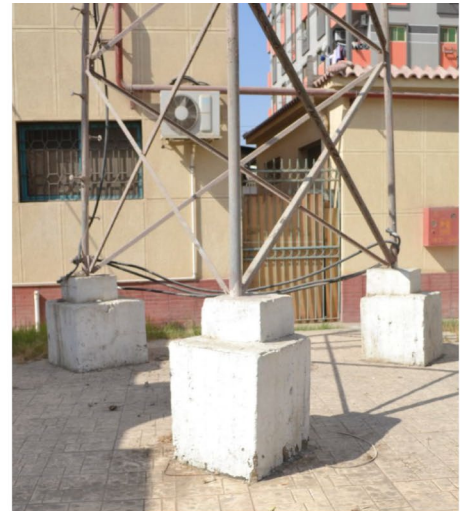
The tower foundations
