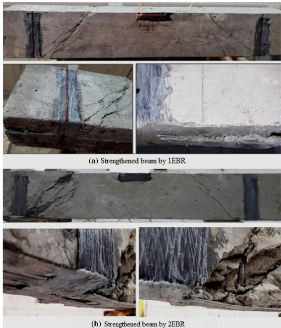
Fig. 6 Failure mode of strengthened beams by EBR technique
