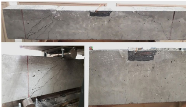
Fig. 5 Failure mode for un-strengthened beam
