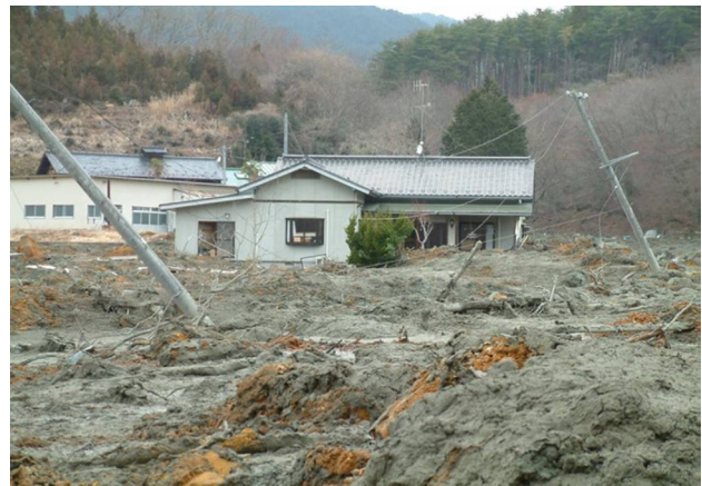
Fig. 12 Affected house inundated by liquefied tailings over the down reach of the Kayakari Stream [114]
