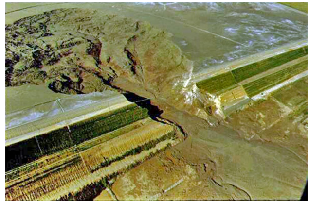
Fig. 7 Aerial view of Merriespruit dam failure [11]
