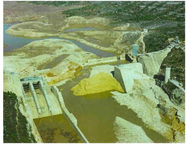
Fig. 6 Tous dam after failure [10]
