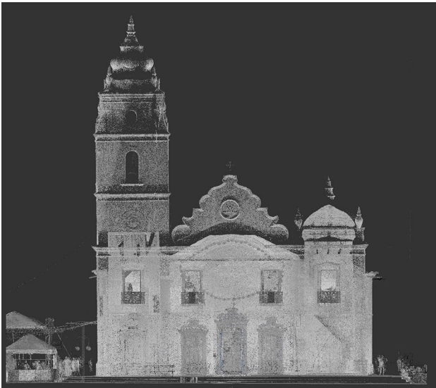
Fig. 7 Front facade of the church
