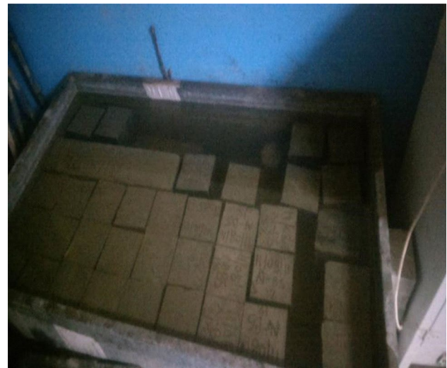
Fig. 6 Curing of concrete
