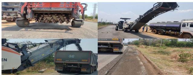
Fig. 6 RAP Extraction process at the field
