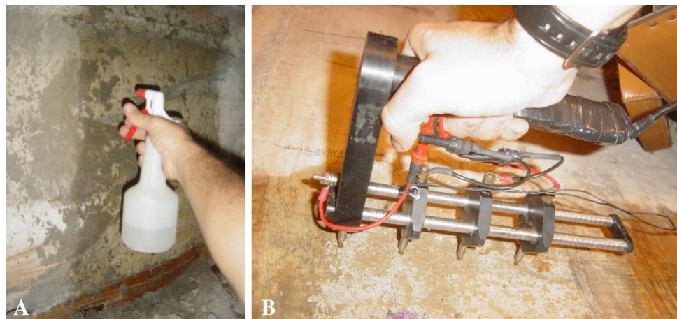
Fig. 6 Electrical resistivity test using the Wenner four-electrode method: a Preliminary wetting; b Apparatus being used on the slab's box void
