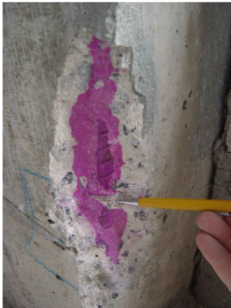
Fig. 9 Carbonation depth test in reinforced concrete inspection work at the Marquee of the Ibirapuera Park
