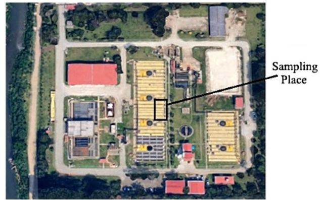
Fig. 2 Layout of Sewage Treatment Station (Source: Google Earth. Accessed on: 12/05/16)
