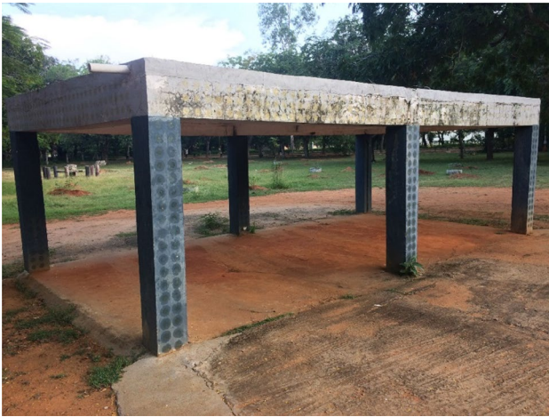
Fig. 3 Photograph of car parking shed located at NITT
