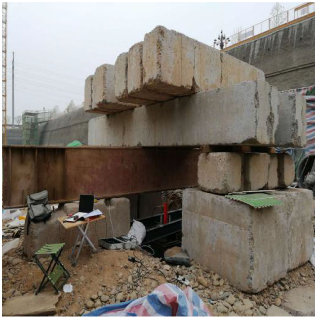
Fig. 6 Test setup for the in situ large-scale direct shear test
