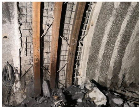
(a) steel arches connected by ribbed steel bar
