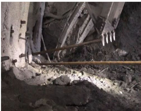
(b) field layout of large lock-foot anchor pipe
