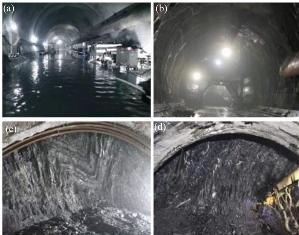
Fig. 5 Underground water condition and surrounding rock structure
