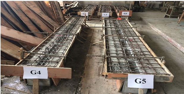
Fig. 13 Preparation of casting the rest of topping slab
