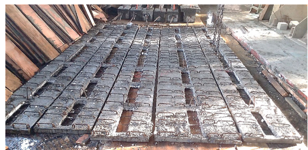
Fig. 11 Lower part of topping slab (precast)
