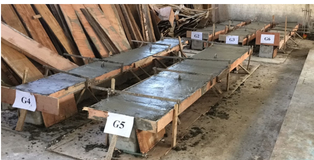
Fig. 15 Finishing casting concrete for the rest of topping slab (G2–G6)
