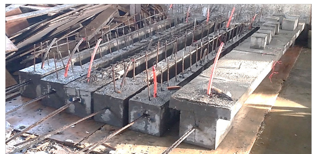
Fig. 10 Control specimen G1 and five girder webs
