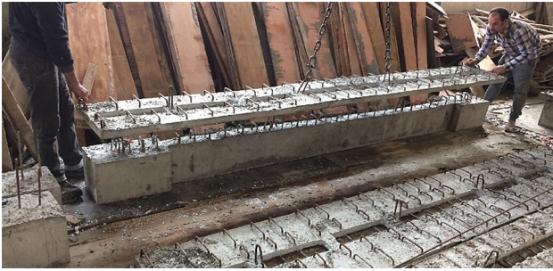
Fig. 12 Installation of the lower part of topping slab above girder web
