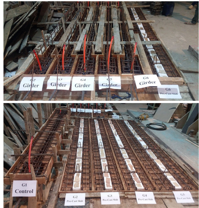
Fig. 9 Finishing preparation of reinforcement for all specimens
