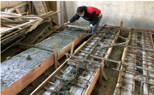
Fig. 14 Casting concrete for the rest of topping slab (G2–G6)
