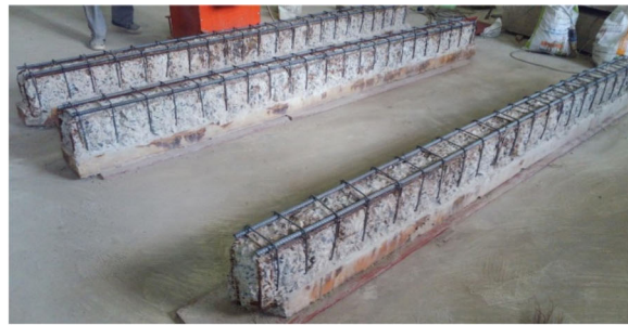
(b) Installing strengthening reinforcing bars
