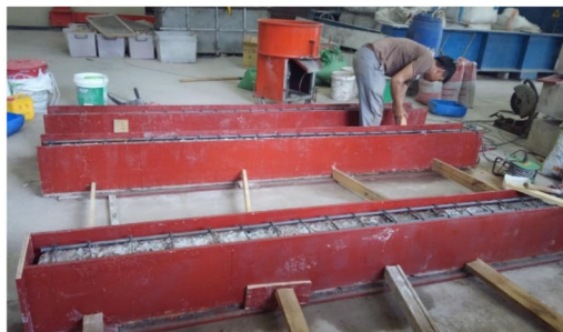
(e) Installing the formworks
