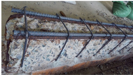
(c) Attachment of new reinforcements
