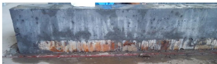
(g) Removing the formworks
