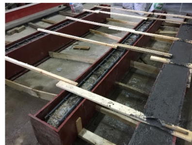
(f) Pouring the high-performance steel fiber mortar
